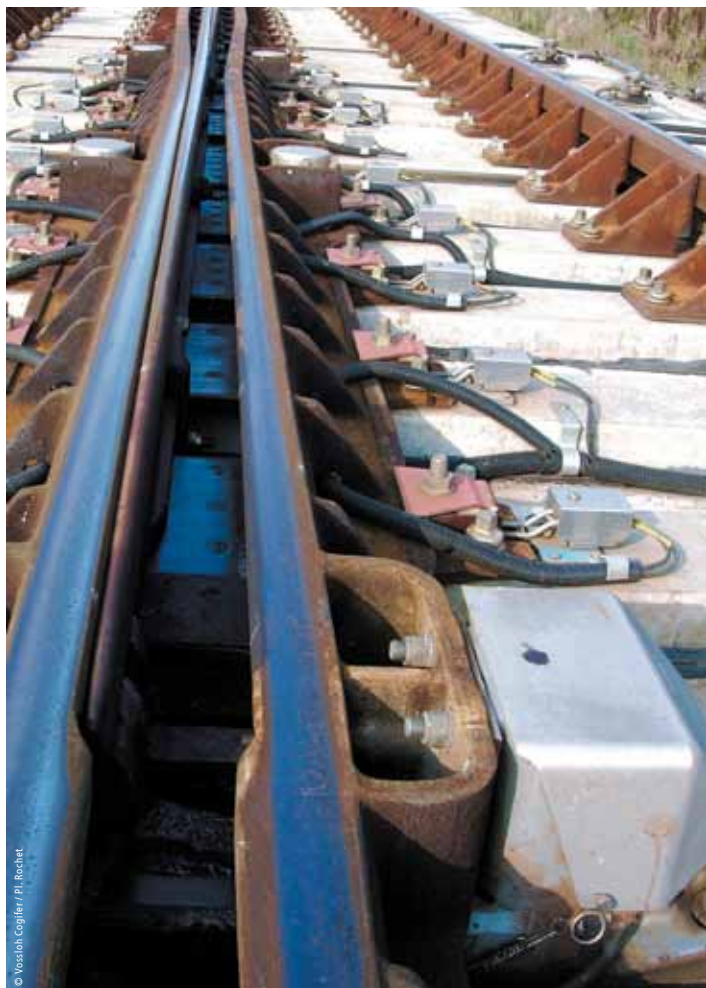
Mobile point lock, East European high-speed line, France
