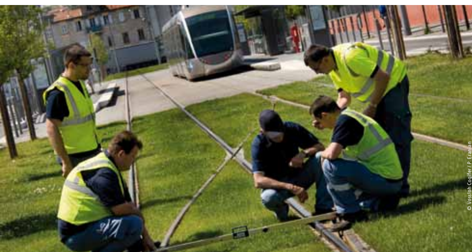
Geometric assessment of a point and crossing, Nice, France
